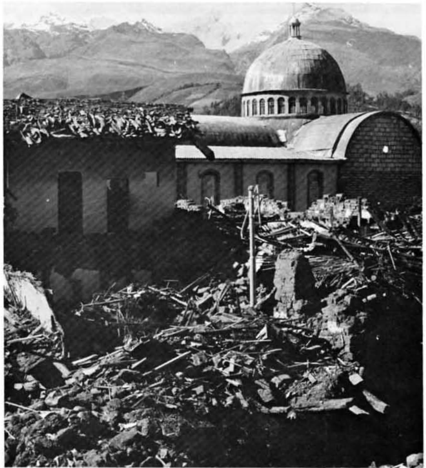
Above: An indication of the damage wrought by the Peruvian earthquake. Over 70,000 were killed in a few hours.
